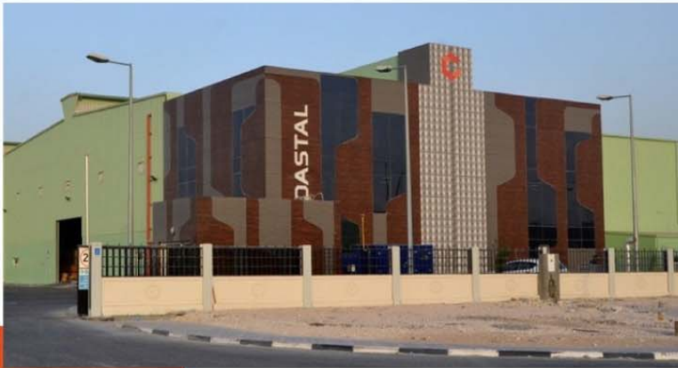
Hot Dip Galvanizing & Injection Molding Plant
